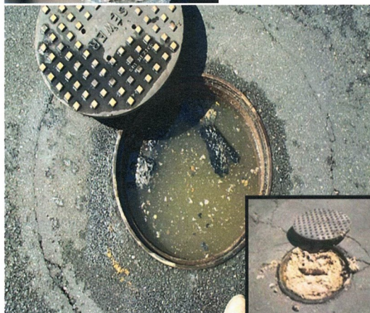
The sewer pipe (above) is blocked by grease buildup.
